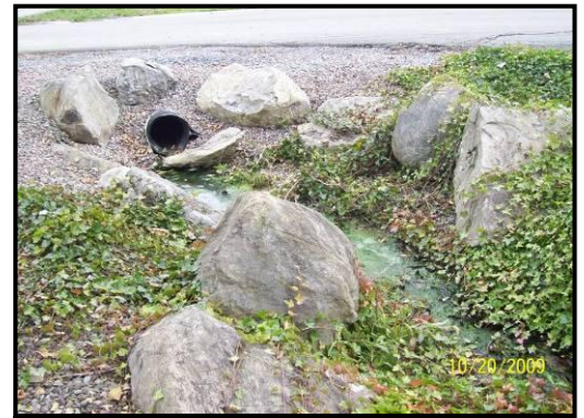
Green residue within ditch is algae. Excessive nutrients are being deposited, causing the algae to grow.
