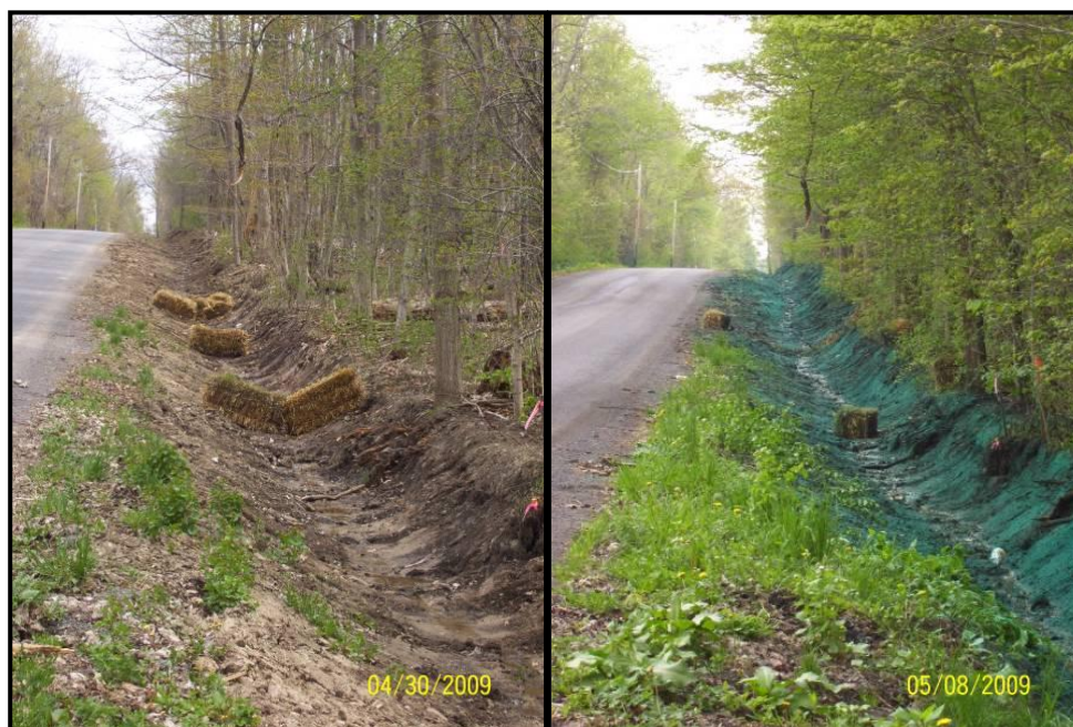
Before and after of roadside ditch that was hydroseeded by the Cayuga County SWCD in order to reduce erosion, establish vegetation to filter nutrients, and slow the flow of water in the ditch.
